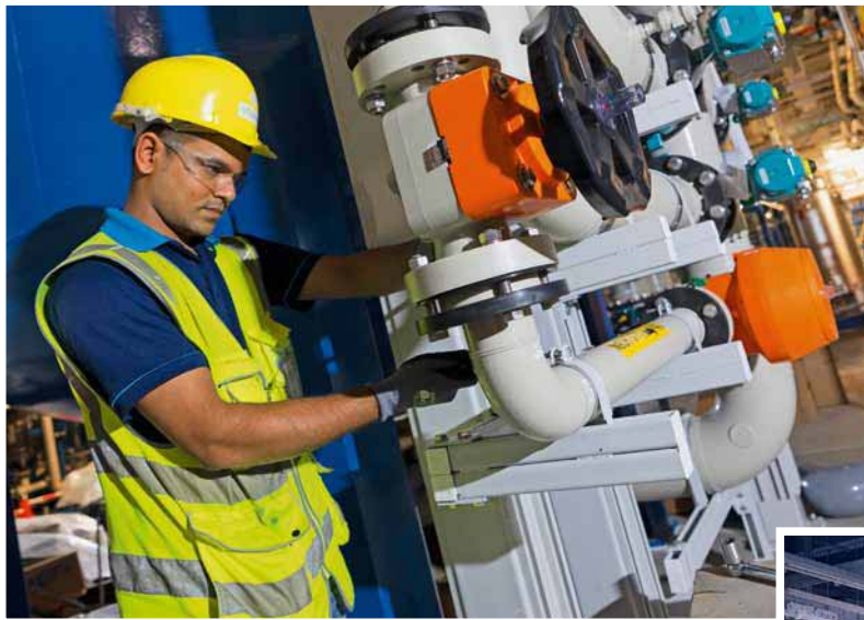
SYGEF Plus in action: The system of pipes, valves, and measuring instruments carries highly sensitive processing fluids safely around the Micron cleanroom facility. (Top right; f.l.) Elin Teo, Jo Lim, and Ramesh Dhanabalan, Global Facilities, Construction & Engineering, Senior Manager at Micron, are all very proud of the result.
