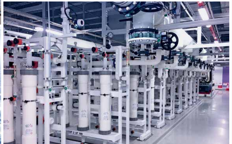
SYGEF Plus in action: The system of pipes, valves, and measuring instruments carries highly sensitive processing fluids safely around the Micron cleanroom facility. (Top right; f.l.) Elin Teo, Jo Lim, and Ramesh Dhanabalan, Global Facilities, Construction & Engineering, Senior Manager at Micron, are all very proud of the result.
